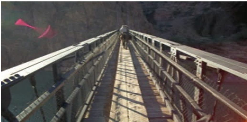
Crossing the Colorado River on the suspension bridge
