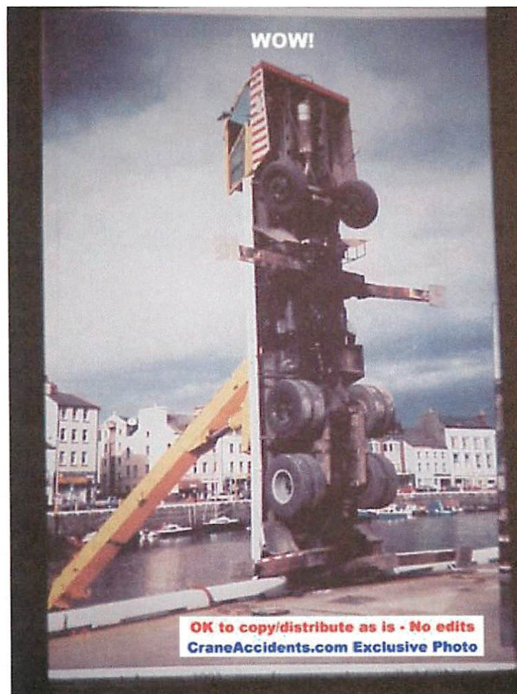
Crane Tipped Forward
