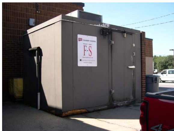
Exterior Walk-in Freezer
