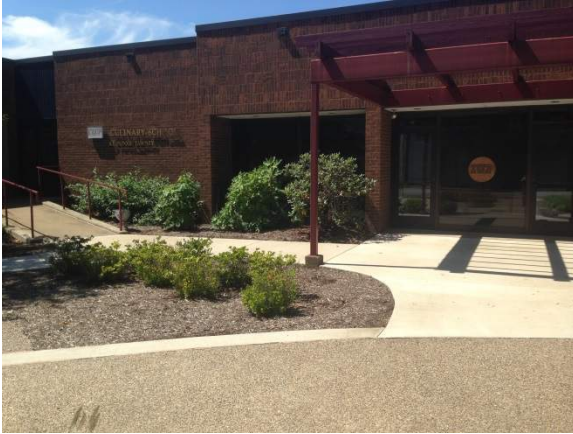
View of Main Entrance (East Side of Building)
