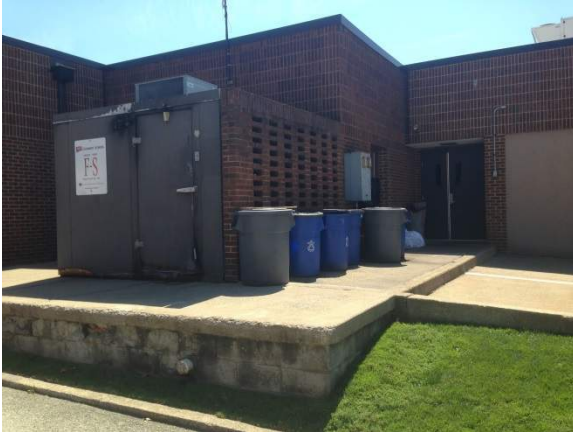
View of Loading Area and Walk-In Cooler from North
