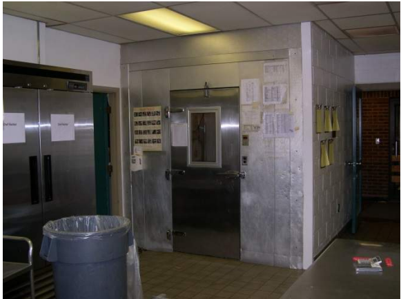
Existing Walk-In Cooler
