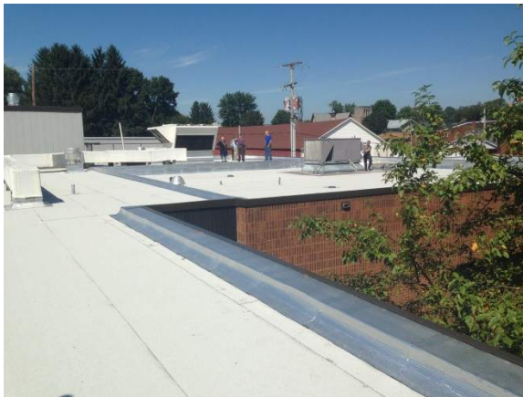
View of Roof, Facing Northwest
