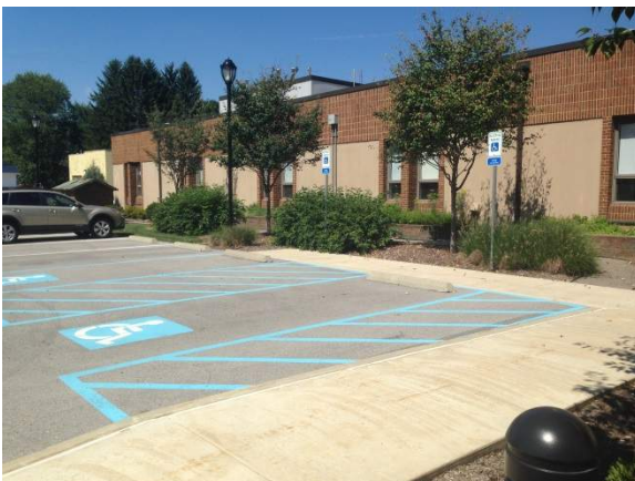
View of ADA Parking on South Side of Building
