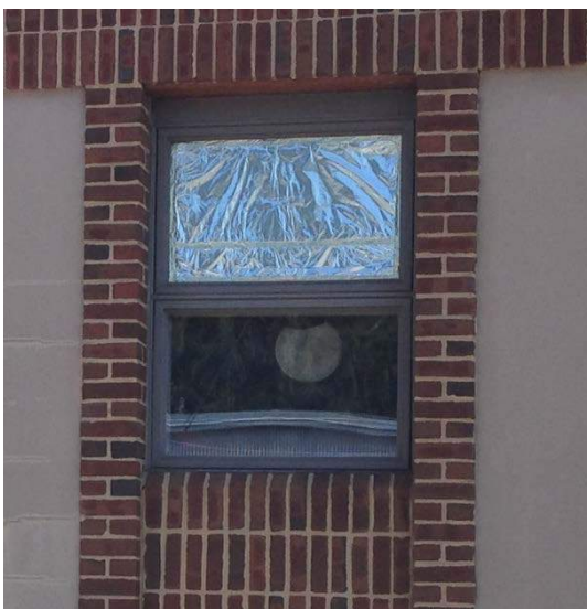
Foil on Kitchen Windows, View from Exterior
