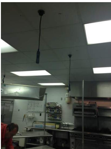
View of Typical Instructional Kitchen
