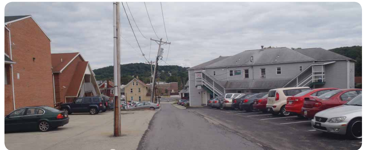
Development patterns in older student housing areas are visually cluttered, disorganized, and lacking in open space.
