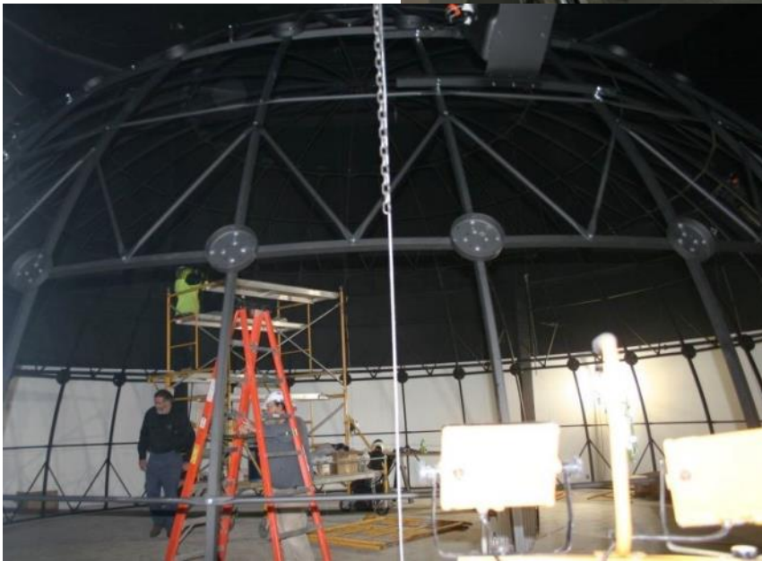
The framework that will support the dome in the Cejka Planetarium has been assembled and is ready to hoist into place for mounting of the dome surface.
